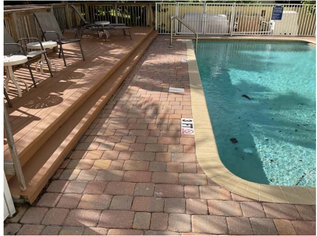
Paver pool deck overview
