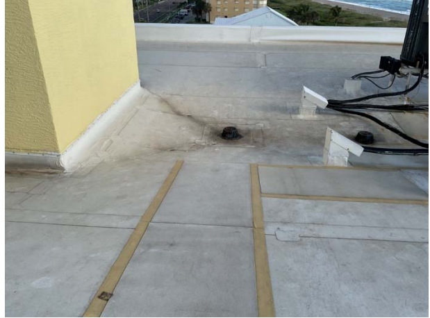
Thermoplastic roof overview
