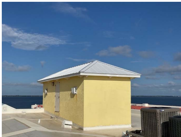
Metal roof at the north elevator room
