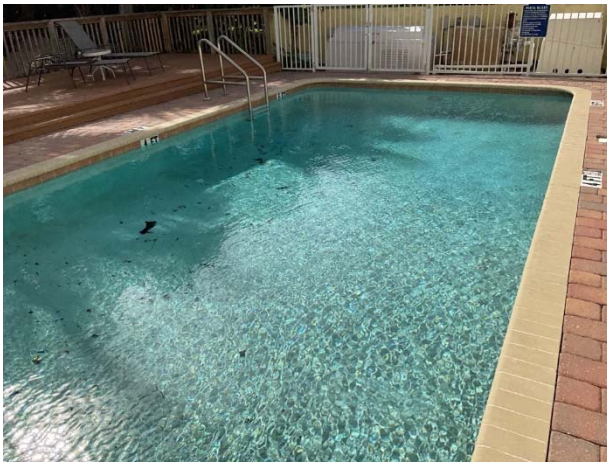
Pool plaster finish with tile perimeter
