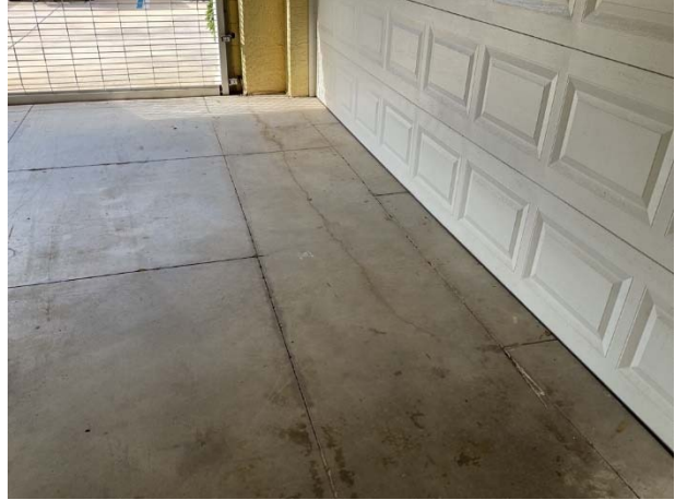
Concrete cracks
