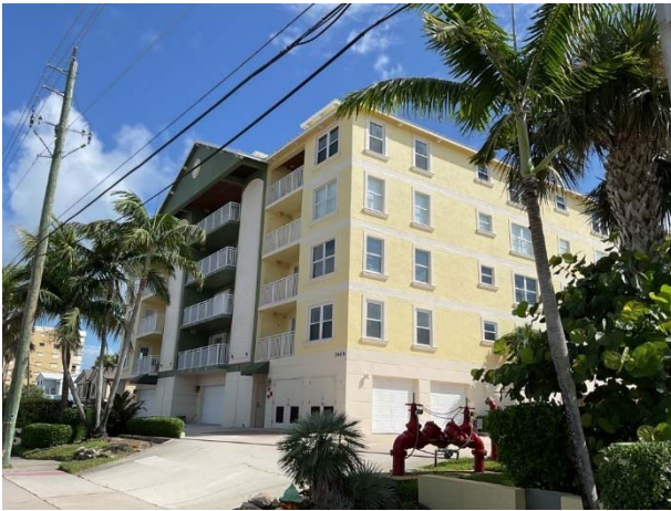
Exterior building overview
