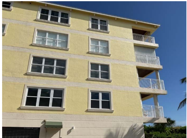
Stucco wall finishes
