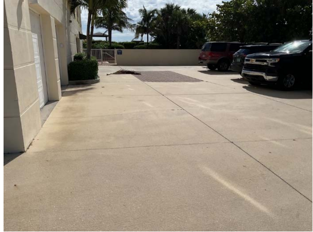
Concrete parking area
