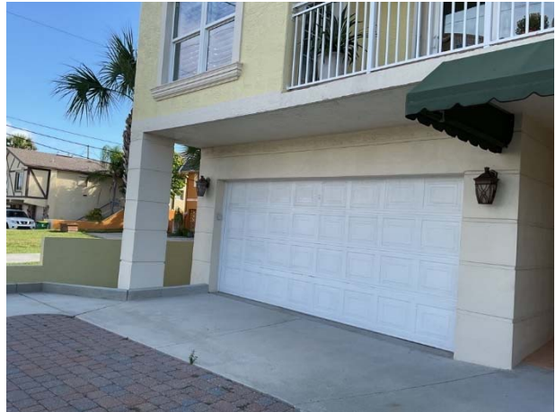
Stucco wall finishes
