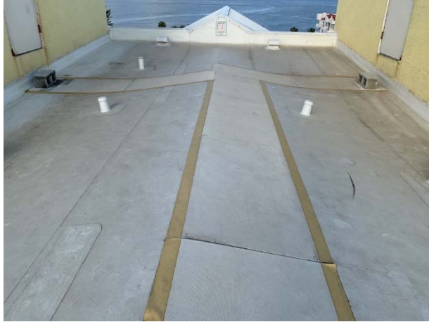
Thermoplastic roof overview
