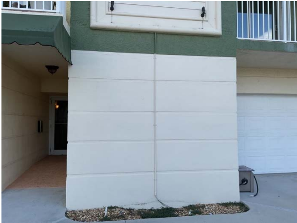
Stucco wall finishes
