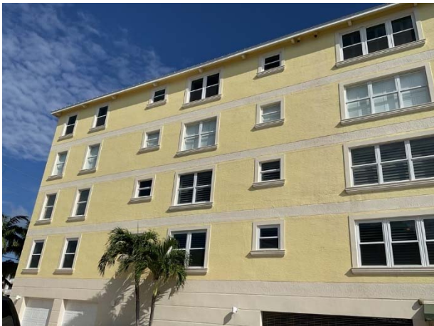
Stucco wall finishes
