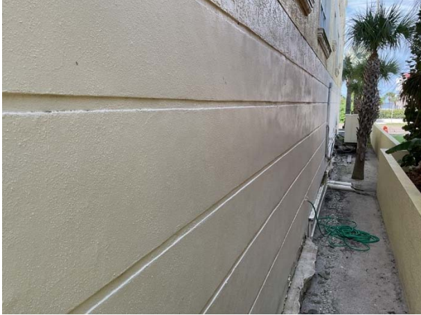
Stucco wall finishes
