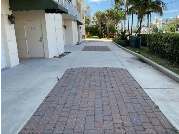
Concrete access drive with paver accents
