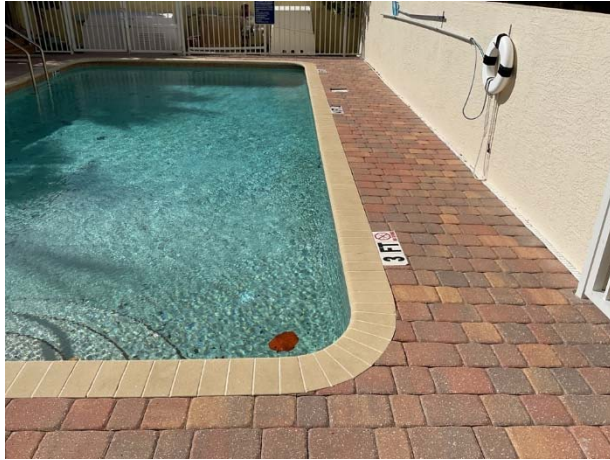
Paver pool deck overview
