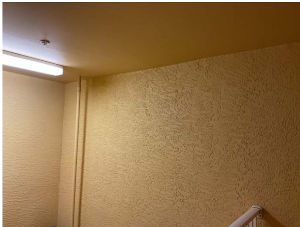
Stairwell paint finishes
