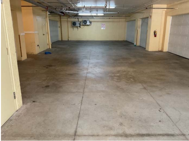
On-grade garage floor overview
