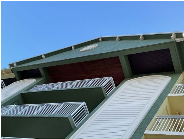
Wood soffit on building front façade
